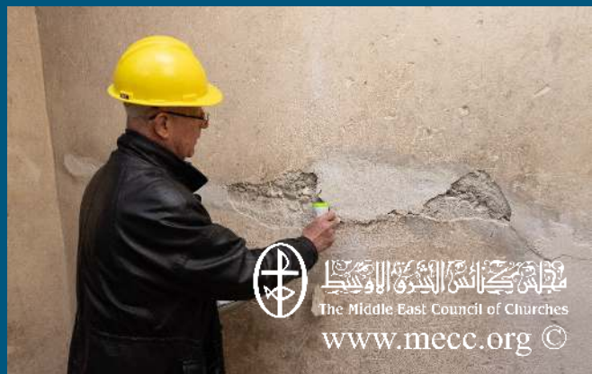
Technical assessments from Engineering teams in Aleppo
