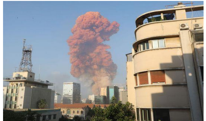
The scene of the blast in Beirut on August 4, 2020. The massive explosion flattened the port silo and several buildings nearby, left 300,000 people homeless and damaged a huge swathe of the city. August 4, 2020, photo credit: Gulf News.
